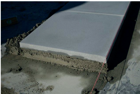
Ideal mortar mix
